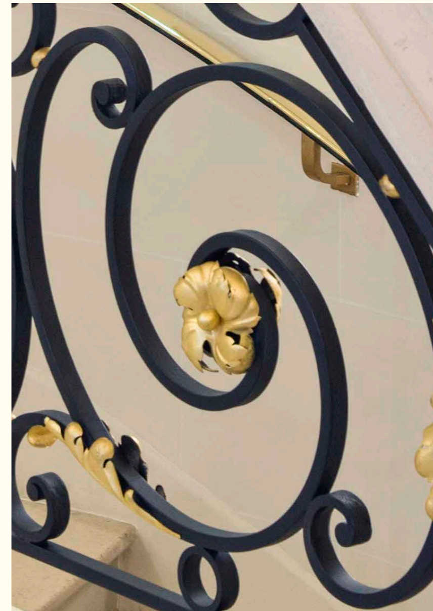
Bannister in soft iron, foliage in sheet metal with gold leaf By Bruno Moinard
